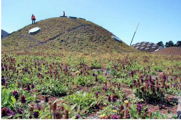
California Academy of Sciences' planetarium dome as seen from its new green roof. California Academy of Sciences photo by Stephanie Stone.
